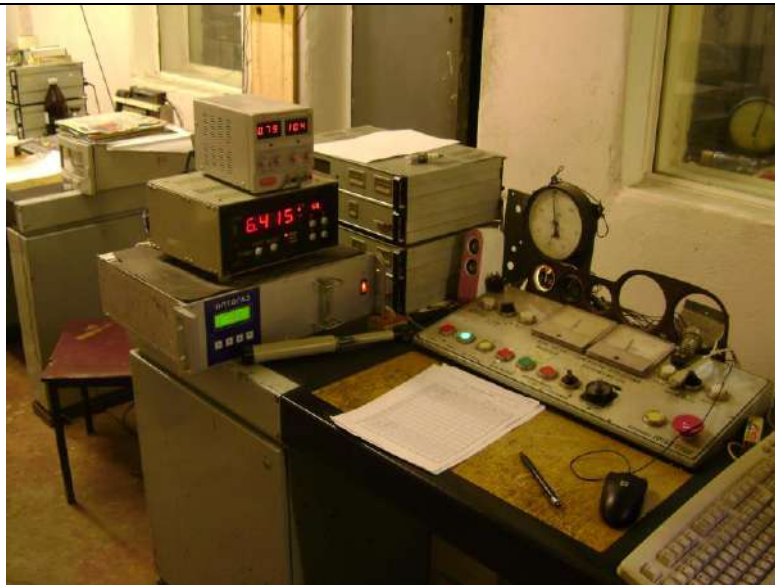
Fig. 3. Control panel. Fuel meter and gas analyzer
