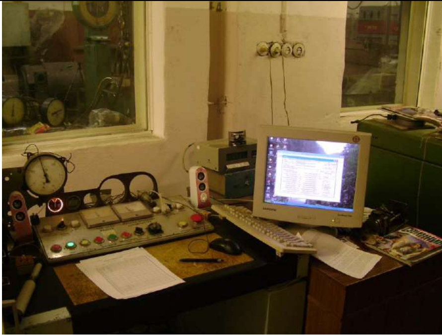
Fig. 4. Control panel. Control console and computerized diagnostic system
